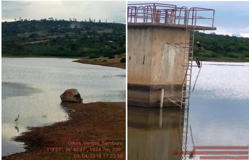
Plate 0-4: Nomotio Dam – the main water supply dam for Maralal Town
