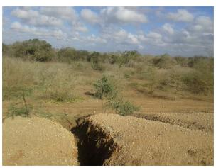
Picture 5-10: Gulley erosion on an unpaved section of the project road
