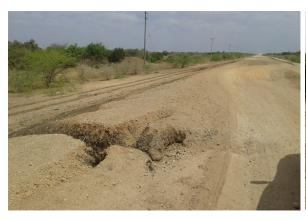
Picture 5-7: Severe soil erosion on the road heading to Hola
