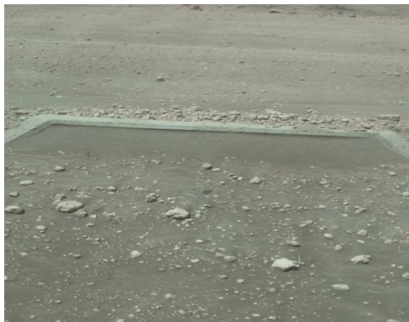
Photo 9.1: Blocked drainage structure along the Lorian Swamp
