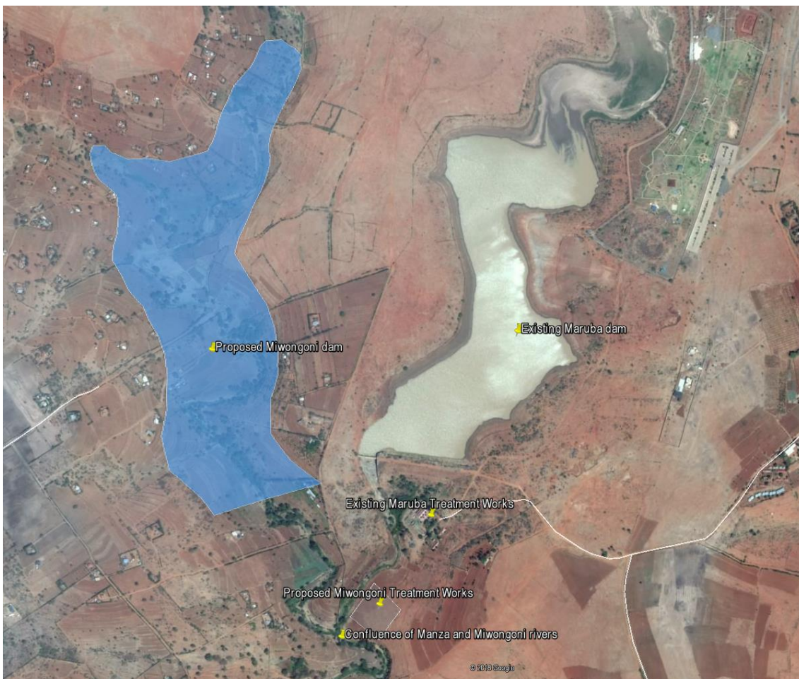
Figure 8-1 Location of the proposed Miwongoni dam and treatment works vs Maruba dam and treatment works
