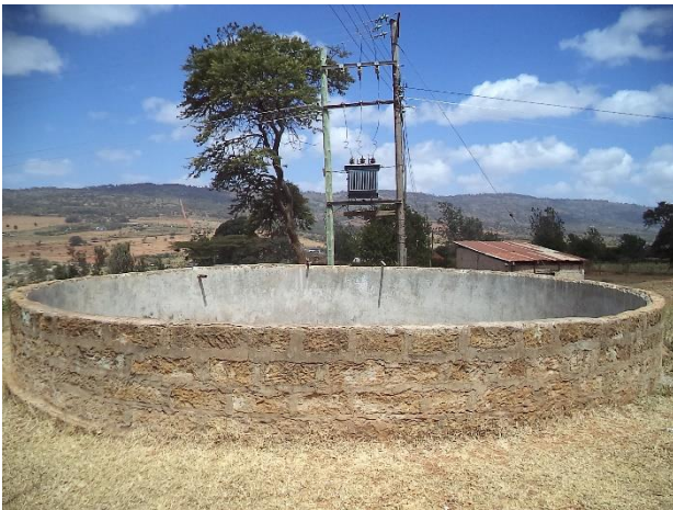
Figure 2-6 Proposed site for Katelembu water storage tank
