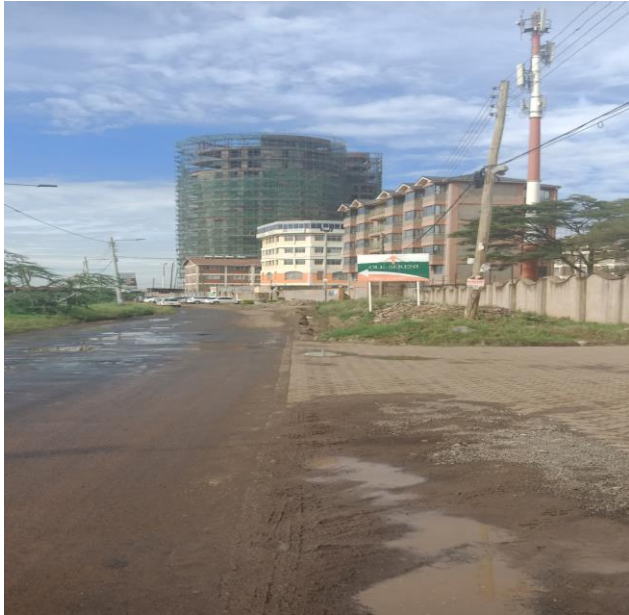
Plate 7; Electricity lines and telecommunication booster
