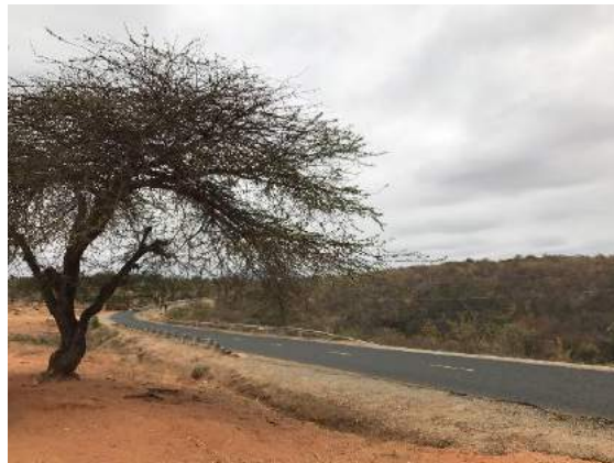
Figure 21: Example B road at point of new access to the site
