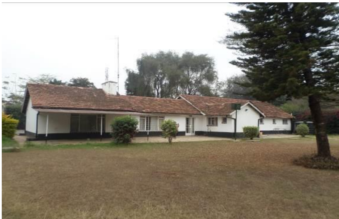
Figure 1: The existing bungalow at the site that will be demolished to pave way for the new multi-storey building
