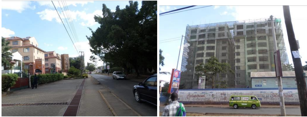
Figure 3: Salonika serviced apartments 4 levels (ground + 3 levels and attic level), apartments 4 levels (ground + 3 levels and attic level) and a 9 storey building under construction bordering the site
