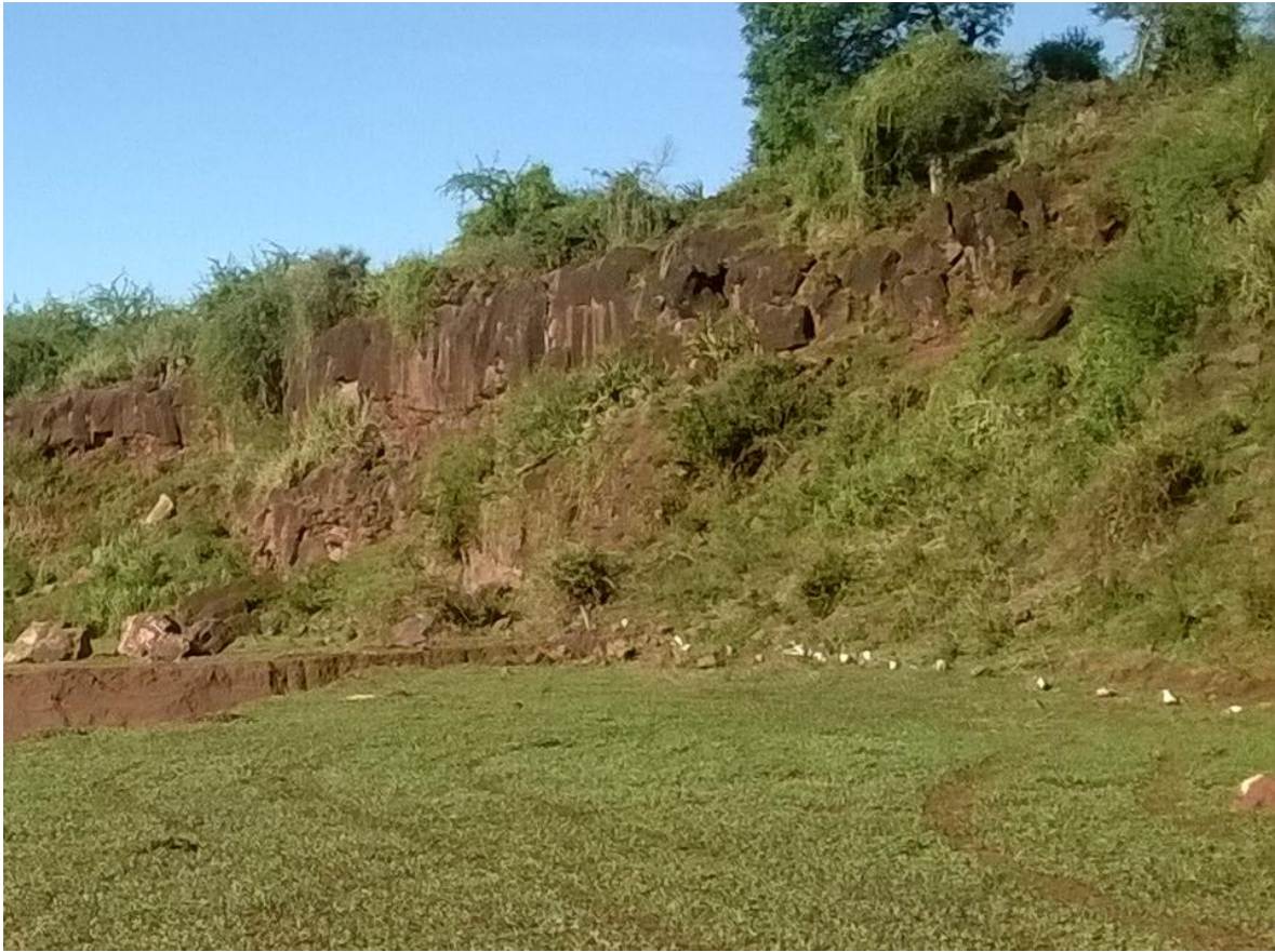
Figure 6:- Basalt cliff on the right bank of Lewa river around the dam axis. The rock exhibits moderate jointing.
