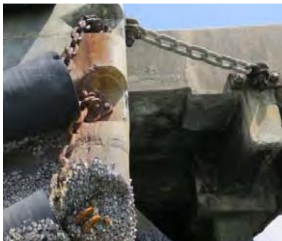
Fig 1.4: Corrosion attack on fenders Berth 11 (Source: Inros Lackner)
