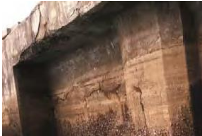
Fig 1.3: Damage to quay wall at Berth No. 9 (Source: Inros Lackner)
