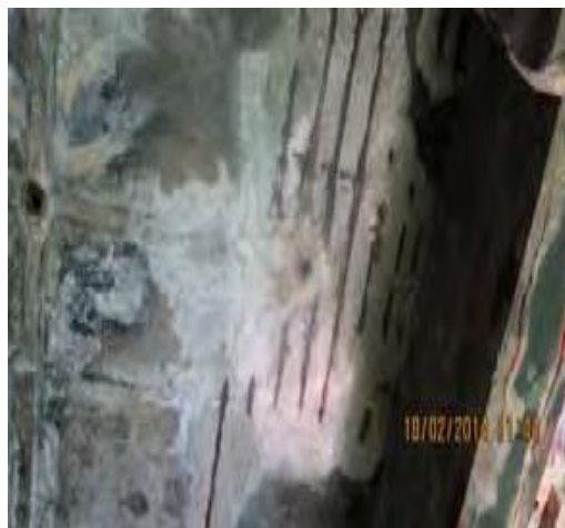
Fig 1.5: Exposed Reinforcement at bottom Berth 11
