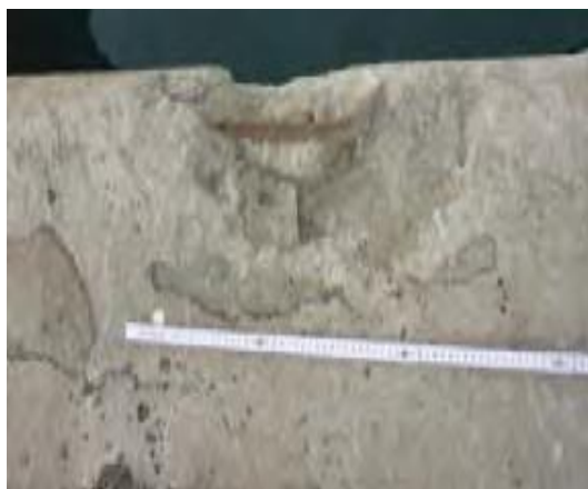
Fig 1.6: Damage to quay beam berth 12
