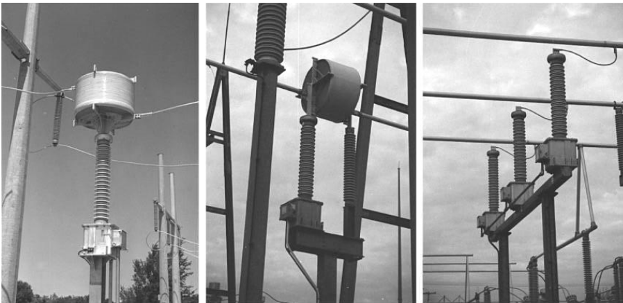
Capacitor Voltage Transformers With and Without Wave Trap. Courtesy of Haefely Trench, Scarborough, Ontario, Canada.
