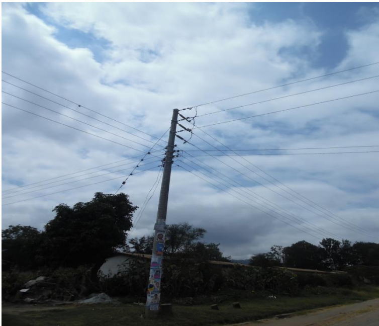
Plate 3: power lines directly opposite the proposed site
