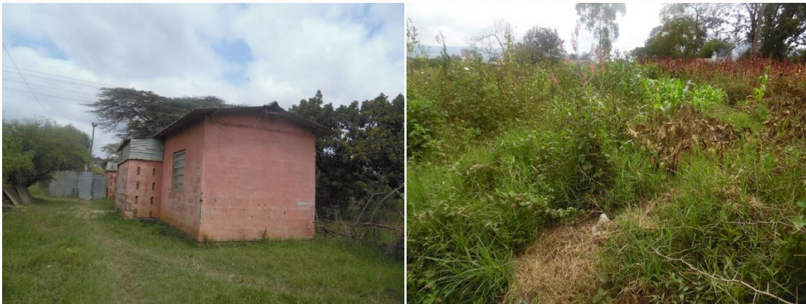
Plate 4: an old house and an idle land for on the proposed site
