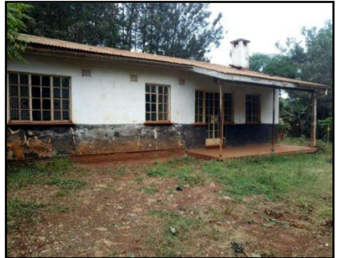
Plate 2: Existing medium grade bungalow
