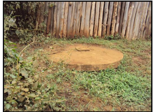
Plate 3: One of the sewer manholes on site
