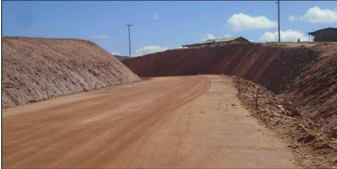
Plate 14: Back Slopes near Chebyamit Market Centre at chainage KM 5+900
