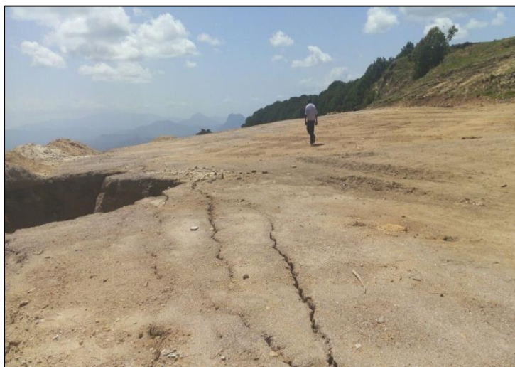
Plate 9: Erosion on a dumpsite at chainage KM 13+100
