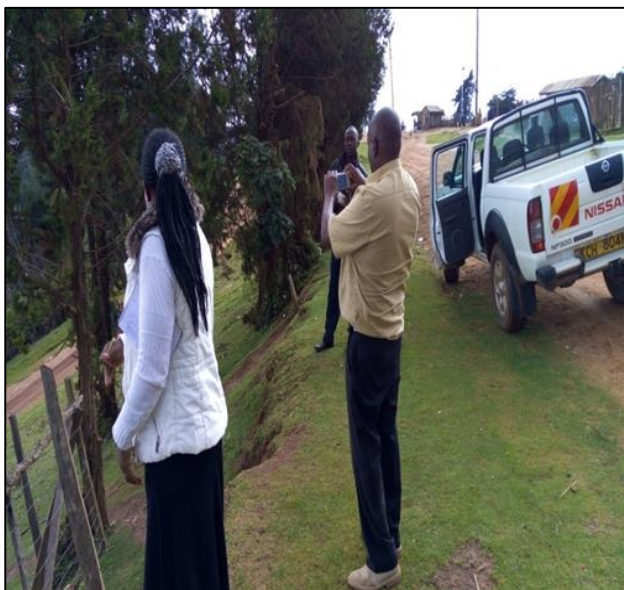
a) Sharp slope – Kimnai on chainage KM 65+100
