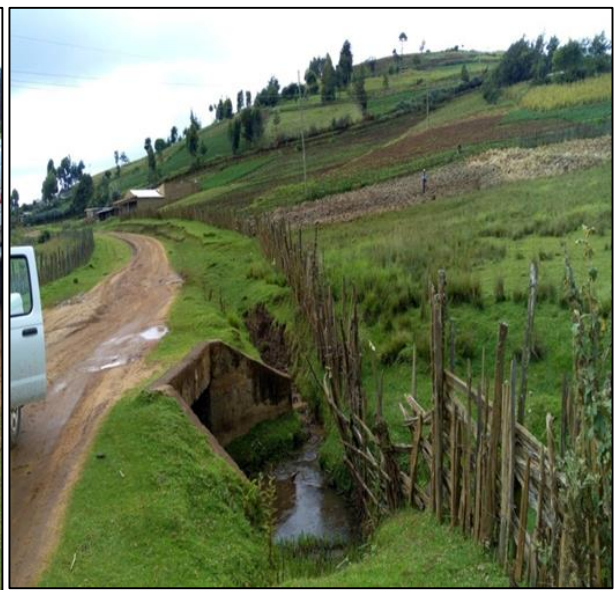
b) Sharp bend – Chebulbai at chainage KM 65+100
