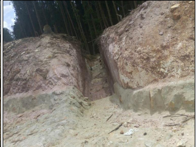
b) An outfall drain into the forest at KM5+400
