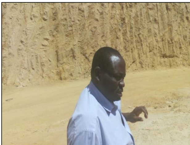
a) Earth works at chainage KM 24+600
