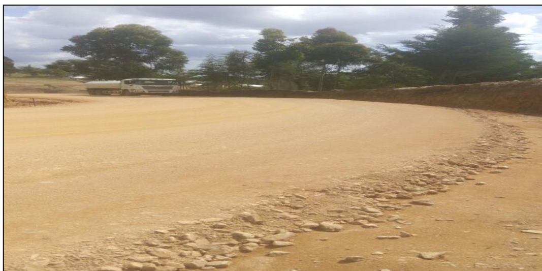
Plate 7: A Very Sharp Curve along the Road at chainage KM 21+620
