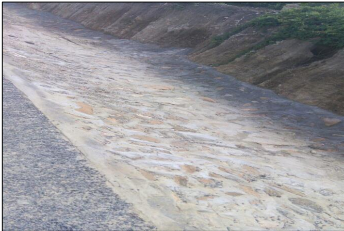
Plate 4: Stone Pitched Area at chainage KM 20+600
