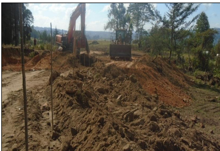
Plate 17: A Diversion under Construction at chainage KM 4+000
