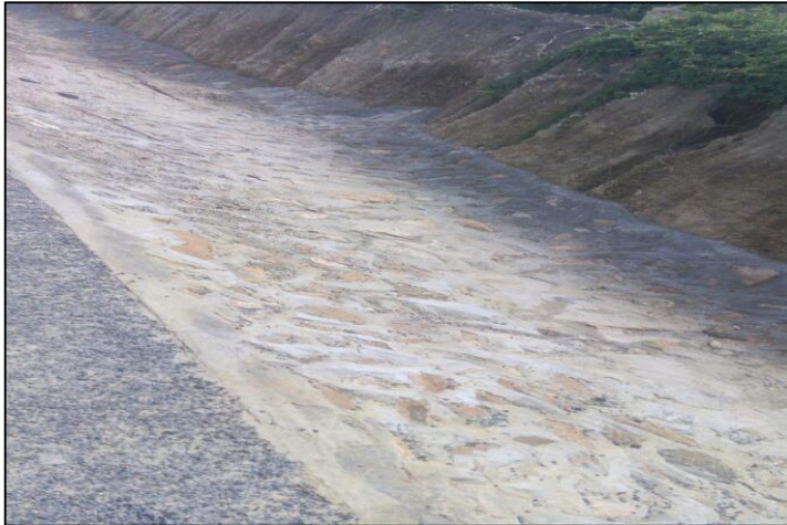
Plate 4: Stone Pitched Area at chainage KM 20+600
