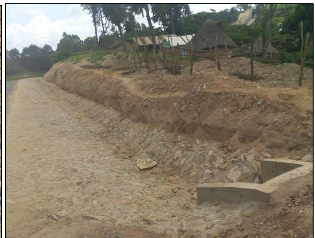
b) Access Culvert under Construction at chainage 21+620
