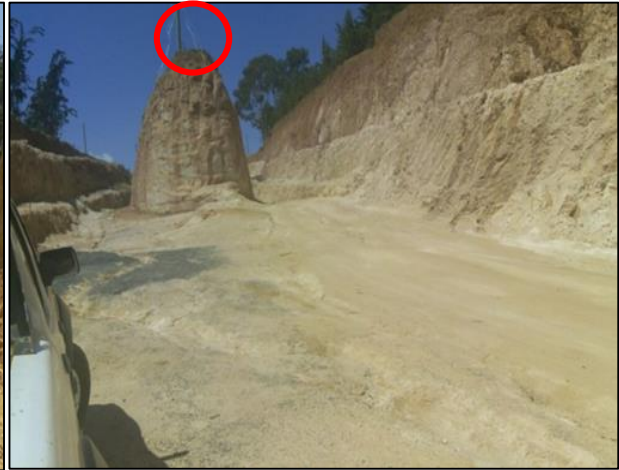
b) Power posts at the middle of the road – see the circle
