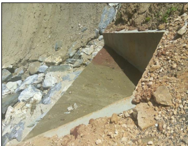
a) Drain under Construction at Chainage KM 1+320
