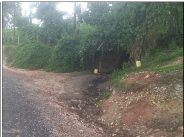
b) An outfall drain into the forest at KM 3+300
