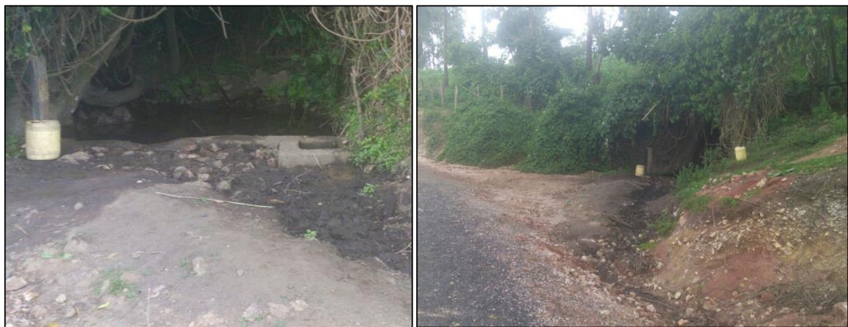
a) A Mitre Drain under Construction at KM 5+800
