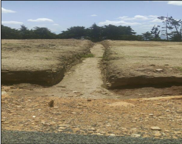
a) A Mitre Drain under Construction at chainage KM 3+300
