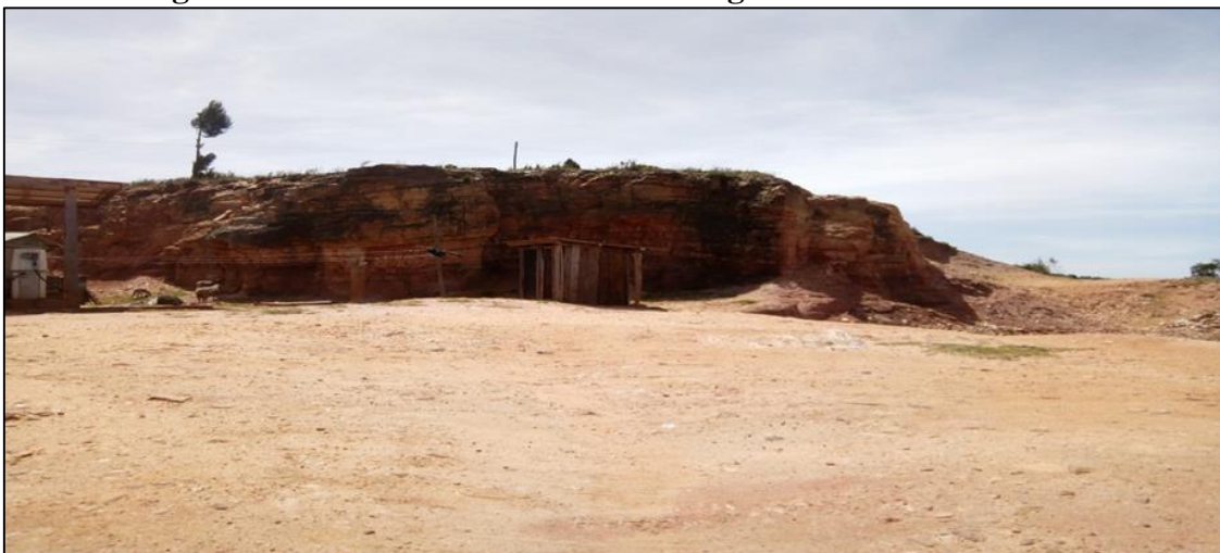
Plate 15: Existing Material Site – Makutano at chainage KM 51+000
