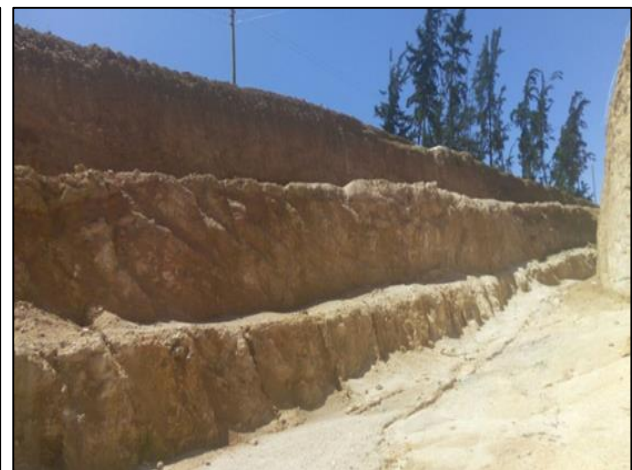
b) Benching on a back-slope at chainage KM 27+200
