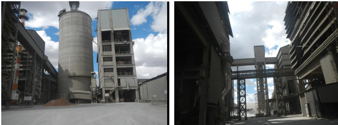
Plate 2: A section of the existing cement grinding mill and silo
