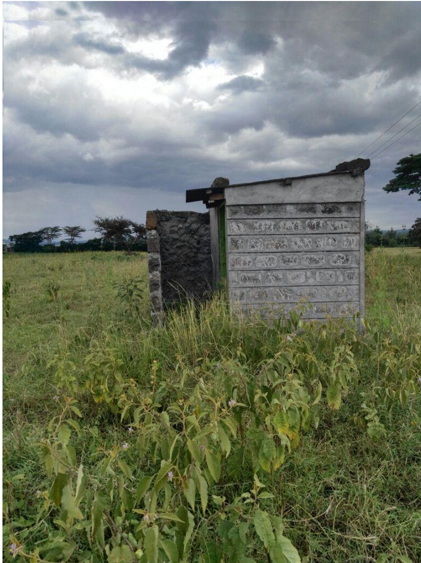
Plate 4: Existing infrastructure on the proposed site
