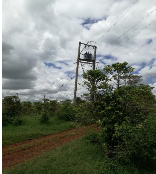
Picture 7: Existing electricity lines through the site
