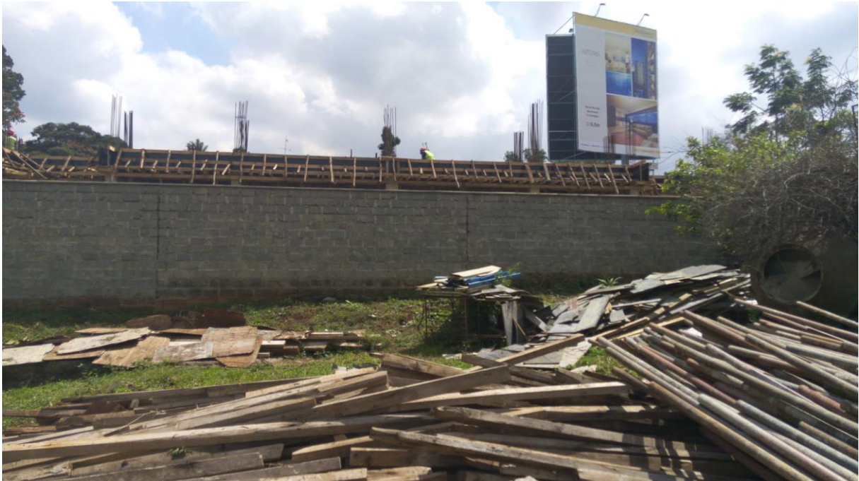
Immediate plot under construction
