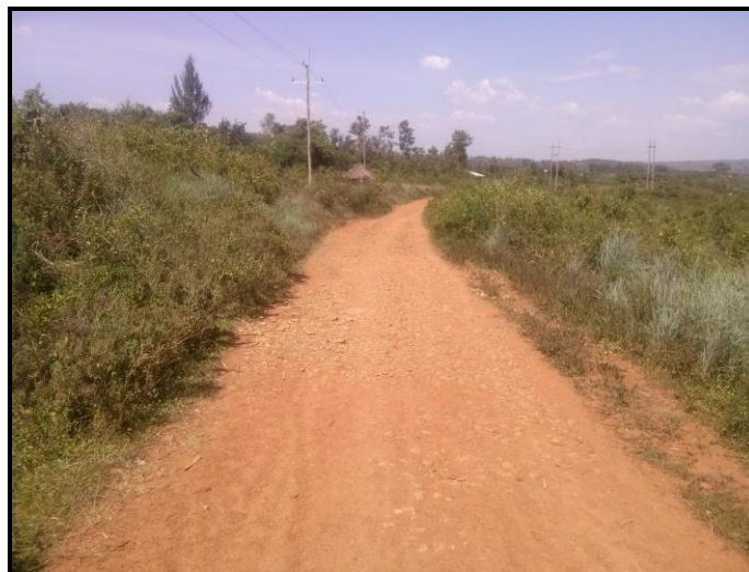
Plate 3: Gravel road traversing the project site
