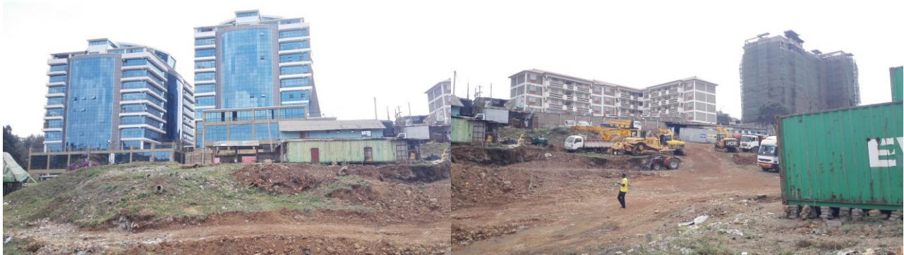
Figure 2; emerging and adjacent developments on site
