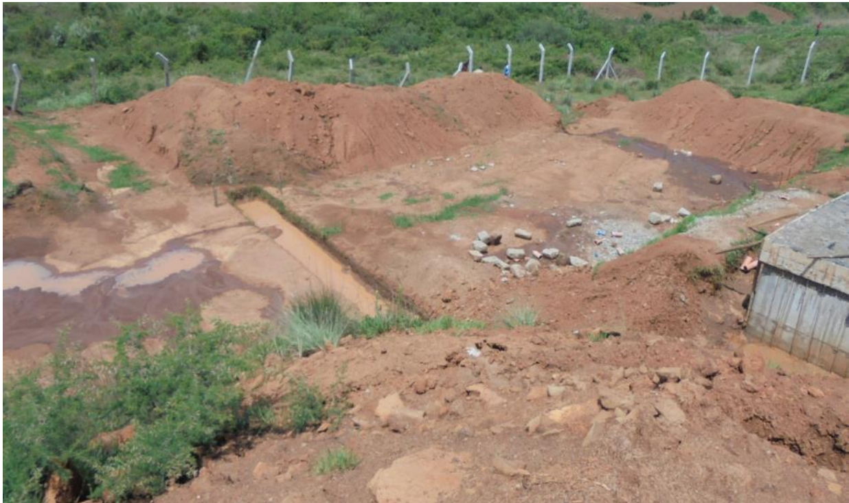
On-going construction of an aerobic treatment facility
