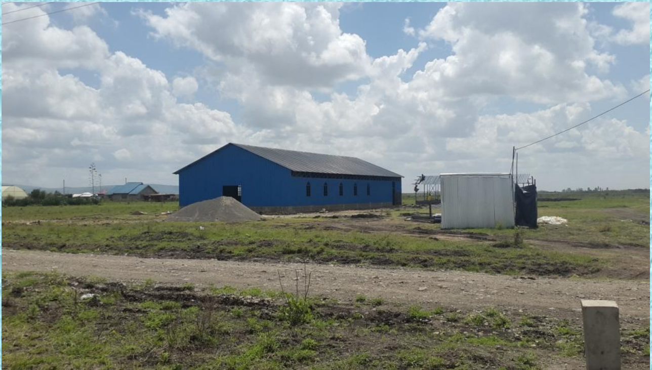
PEFA church under construction directly opposite the project site
