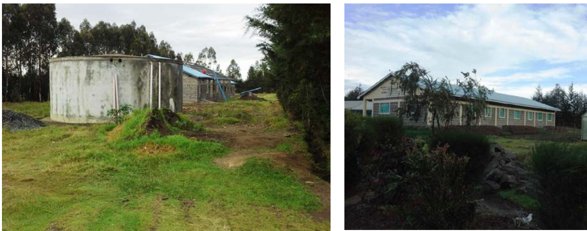
Figure 7.1: Affected structures at Gituru secondary school, Nyandarua county
