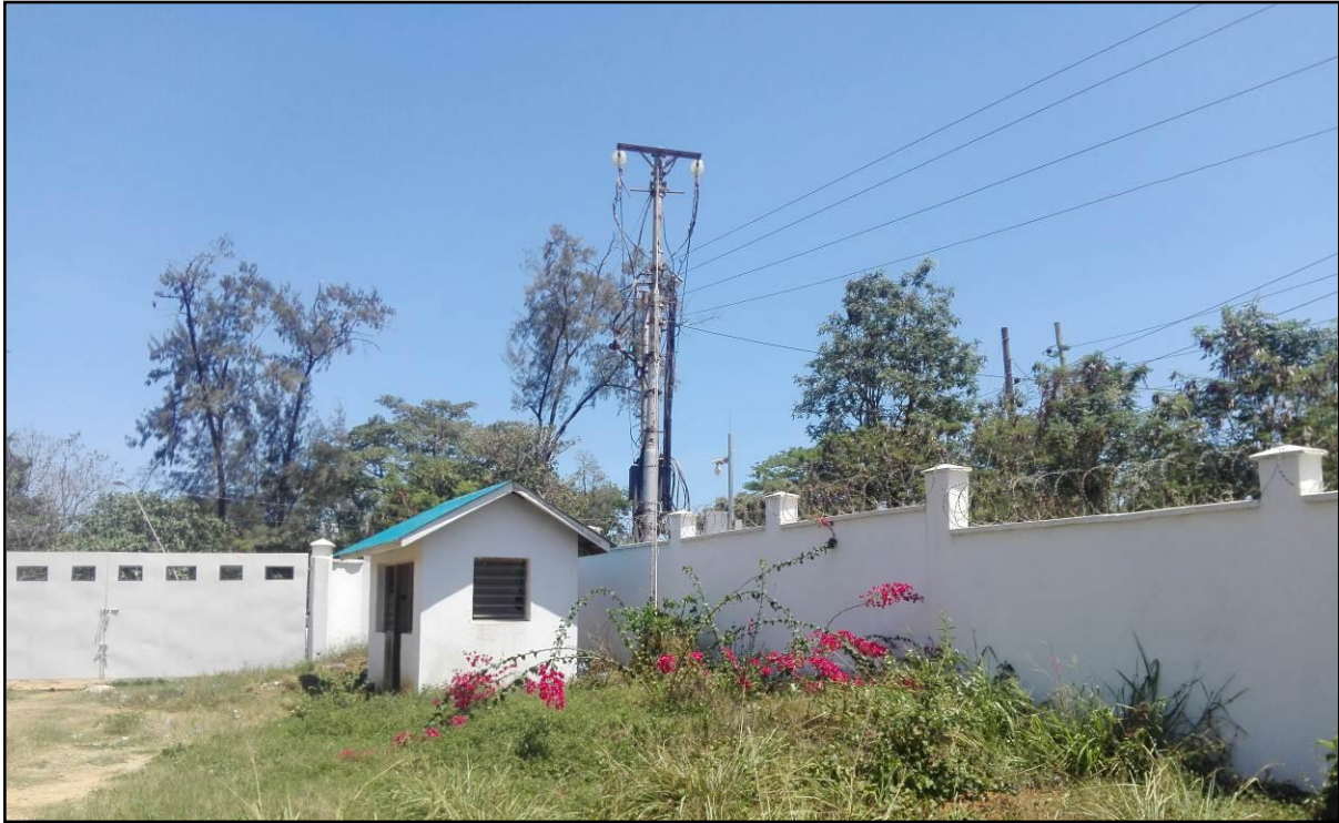
Figure 2.4: A section of the proposed site showing the existing power installation & Boundary wall
