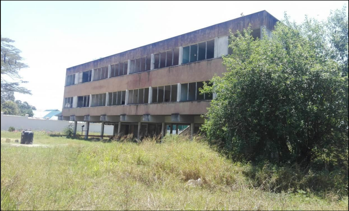
Figure 2.2: The proposed site showing the existing structure to be demolished
