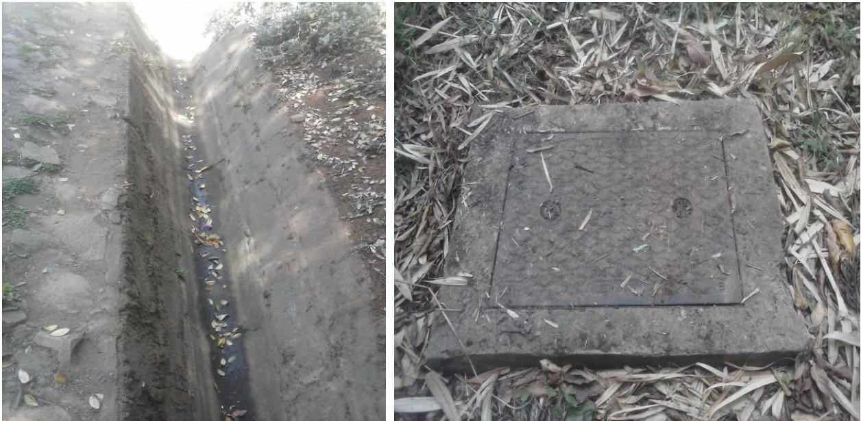
Plate 5: NWSCo manhole and Open Drains along the road
