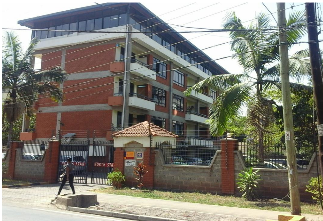
Plate 10: Electrical infrastructure passing along Lenana Road
