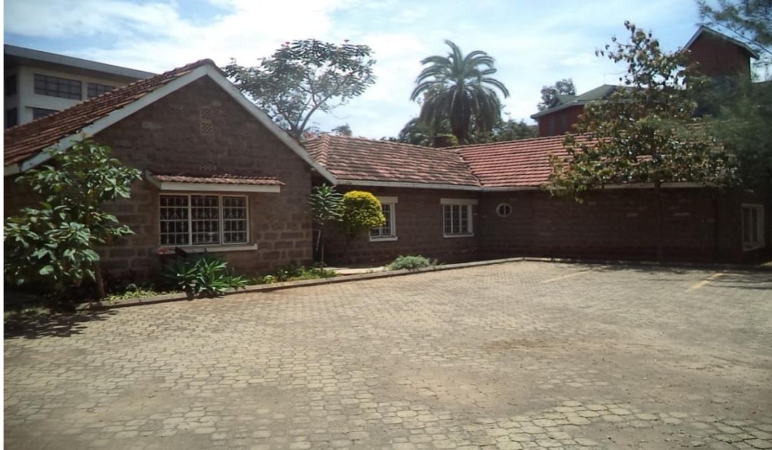
Plate 2: A bungalow on the property set for demolition
