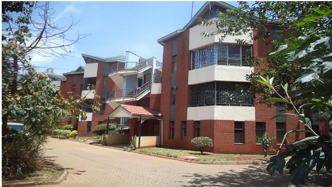
Plate 3: A 3-Storey building on the property set to be demolished
