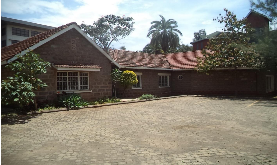
Plate 4: A bungalow on the property set for demolition
