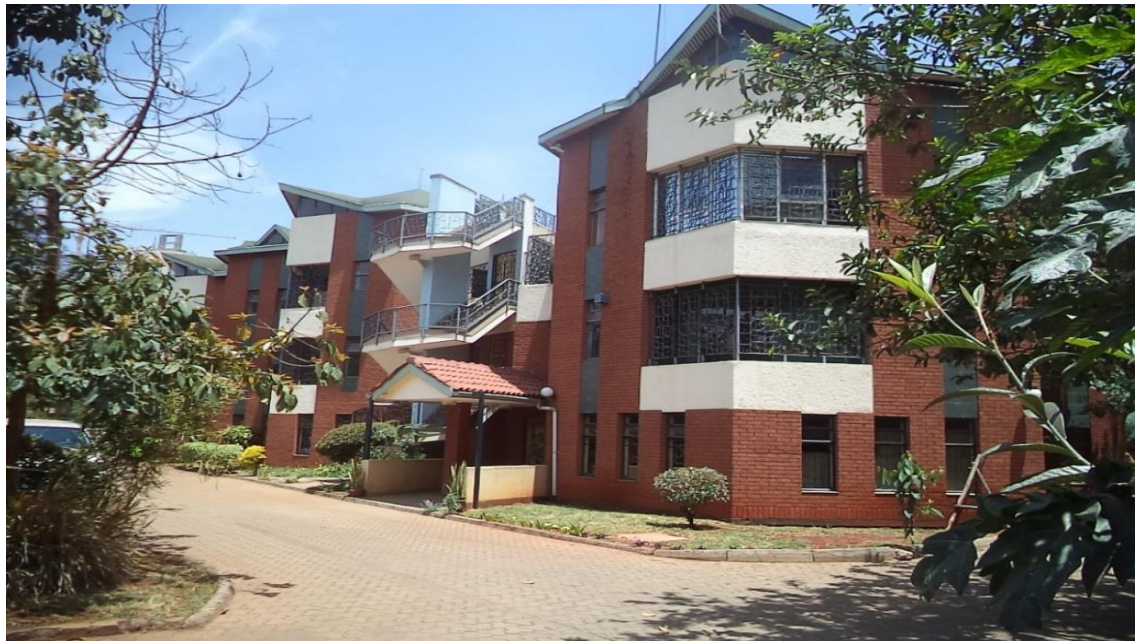
Plate 5: A 3-Storey building on the property set to be demolished
