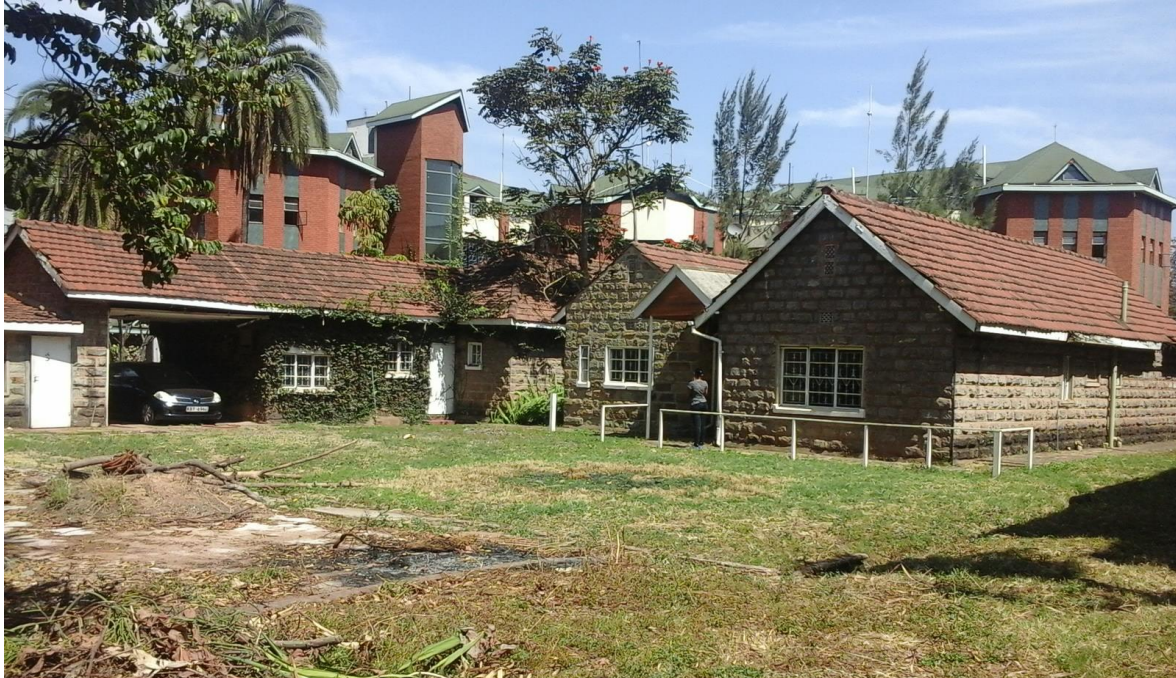
Plate 6: A view from the southern end of the property, of the buildings to be demolished
