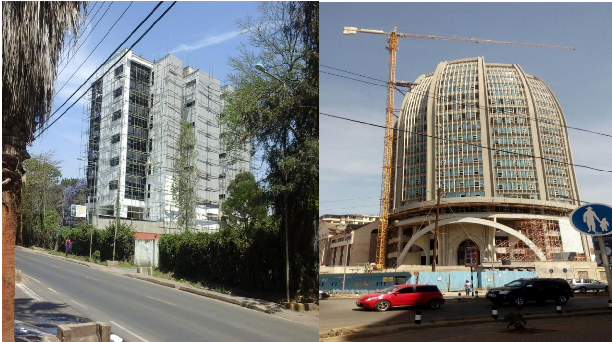
Plate 1: Similar on-going construction projects along Lenana road
