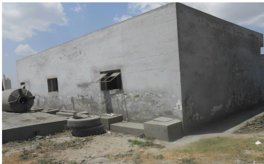
Figure 6: Current worker's washrooms (Likely to be affected)
