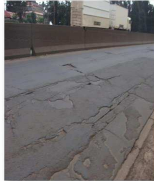
Deterioration of pavement surface
