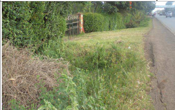
Access to private property lacking access culverts, the home owners cited heavy flooding in their compounds during the rainy season
