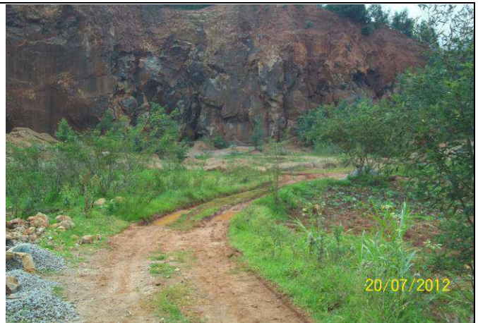
Access road to Kikuyu Quarry, heavy trucks access the quarry likely to impact negatively on this road if prior improvement measures are not considered
