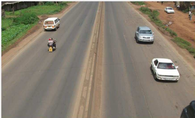
Insufficient margins between New Jersey barriers and traffic lines
