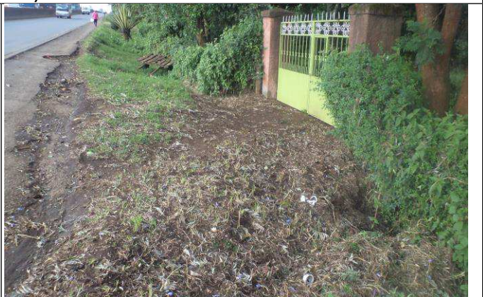
Access to private property lacking access culverts, the home owners cited heavy flooding in their compounds during the rainy season
