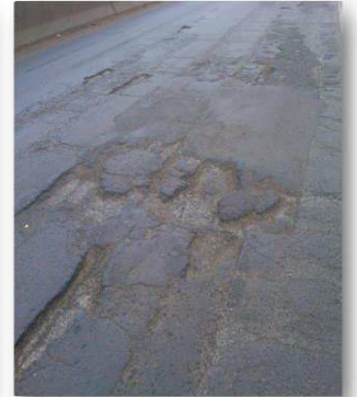
Deterioration of pavement surface
