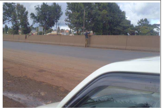
Distant view of a pedestrian crossing at New jersey barrier, this endangers the residents' lives on a day to day basis
