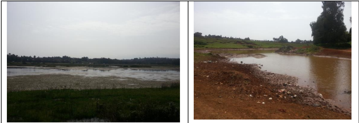
Photo Plate 1: Drainage Basins within Limuru area
