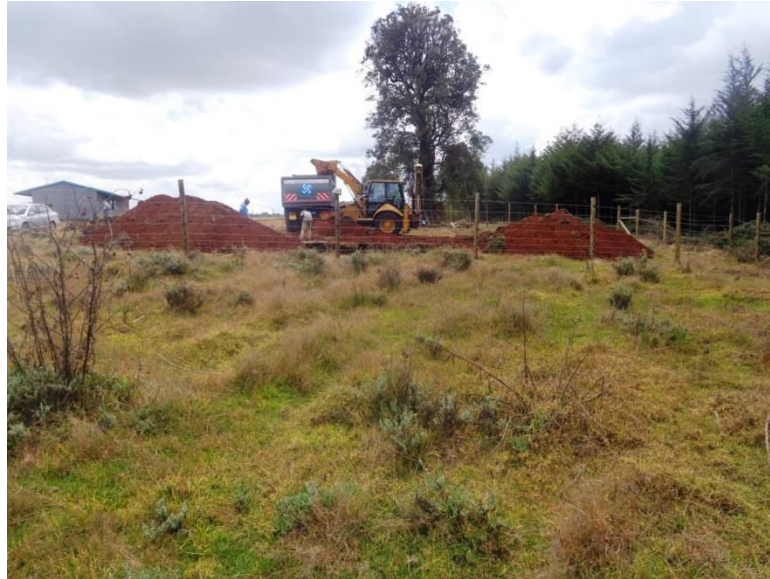
Some excavations and the site office at the background.
