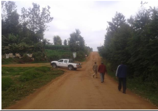
Section of Ndumberi Murrum Road where the sewerline will flow
