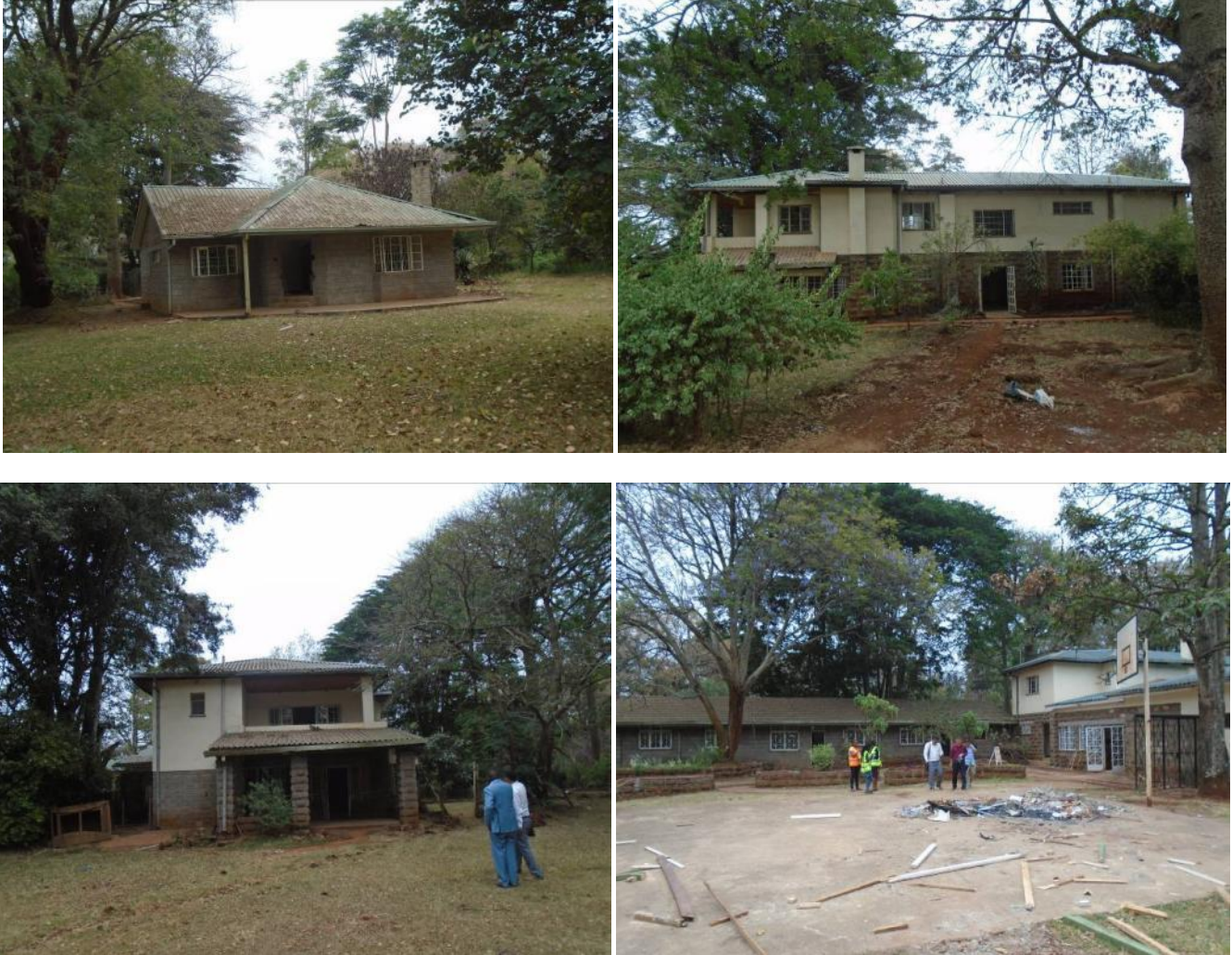
Figure 12: Some of the facilities that will be renovated for use by the construction staff and then will be demolished later
