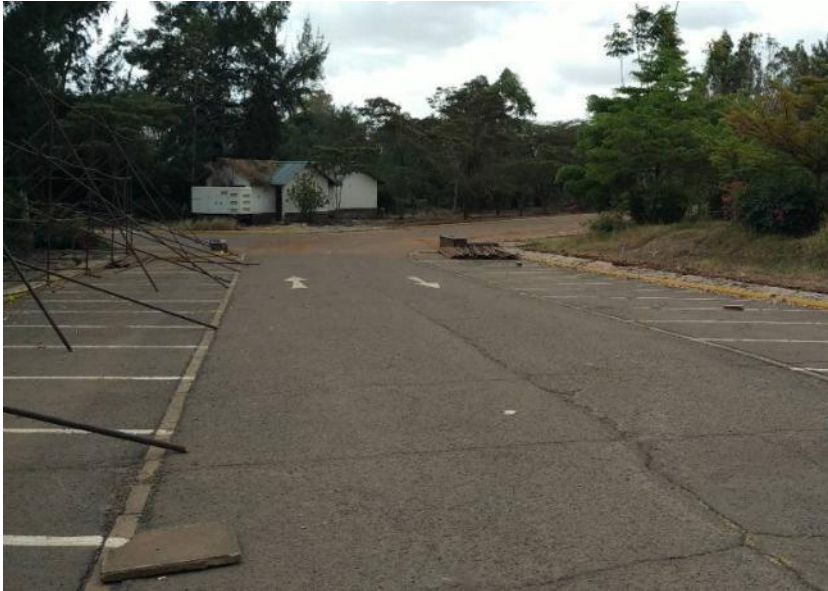
Plate 1: Buildings and road inside the site planned to be demolished.
