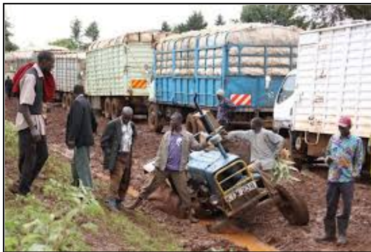
Plate 17: Trucks stuck along the project road in Endebess during rainy season
