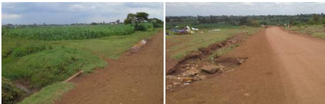
Plate 19: Erosion on the left of the alignment in Endebess area
