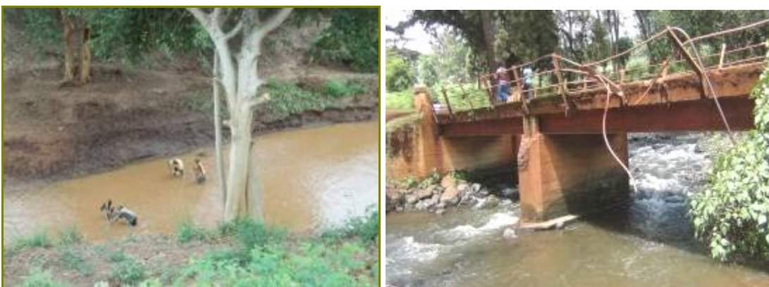
Plate 7: Kaibei River and bridge at 24 km+290 (b) Suam River and bridge at km 45+200
