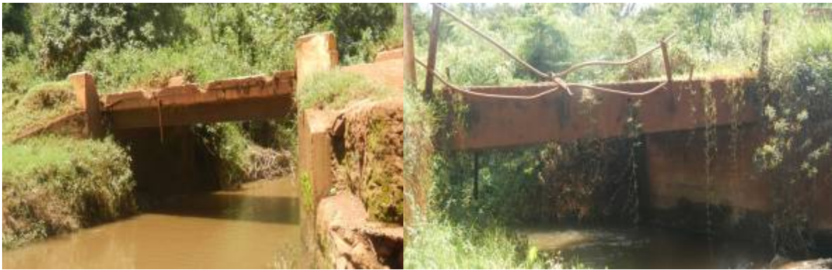
Plate 6: (a) Sabueni River at 20 km +826 of the alignment (b) Mubere River at km 40+477
