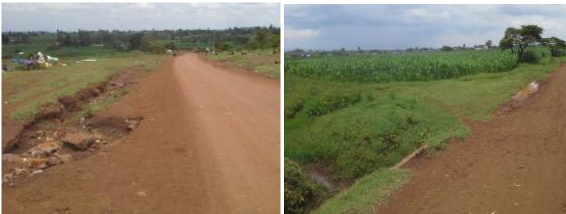
Plate 5: Soil erosion concerns along the alignment in Chepchoina area
